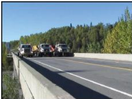
Photos: Load testing of the Chulitna River Bridge's newly installed SHM system. Photo credit AUTC.
