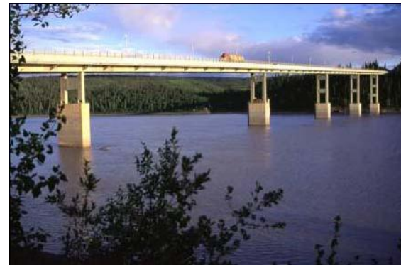
Yukon River Bridge
