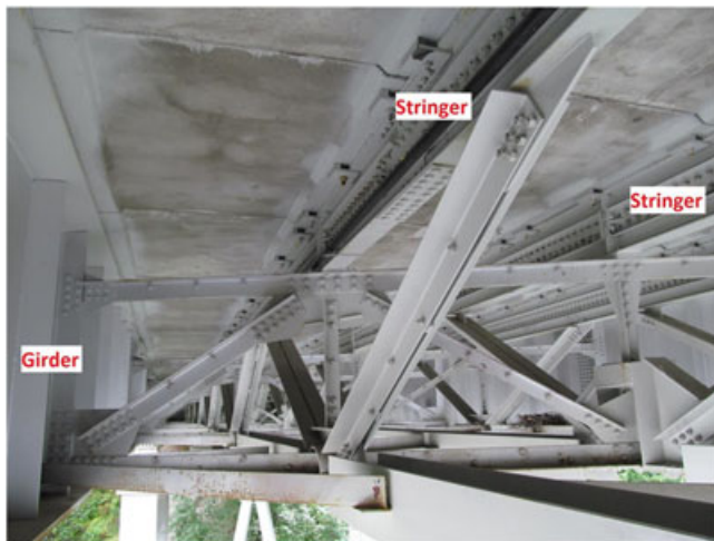
FIGURE 7 Steel-concrete composite condition
